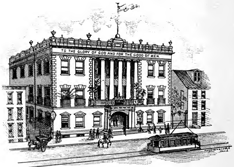
ASSOCIATION BUILDING, MAUCH CHUNK, PA.
